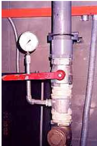
Bourdon pressure gauge to measure pressure of fluid in a pipe.
