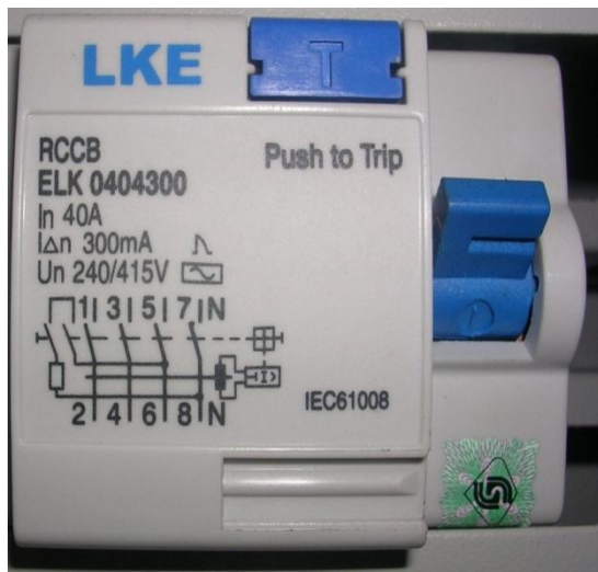
RCCB – INSIDE A DISTRIBUTION BOARD
