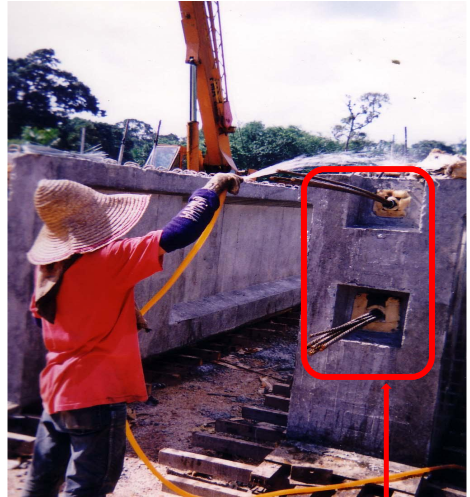
Multi strand tendon live-end anchor
