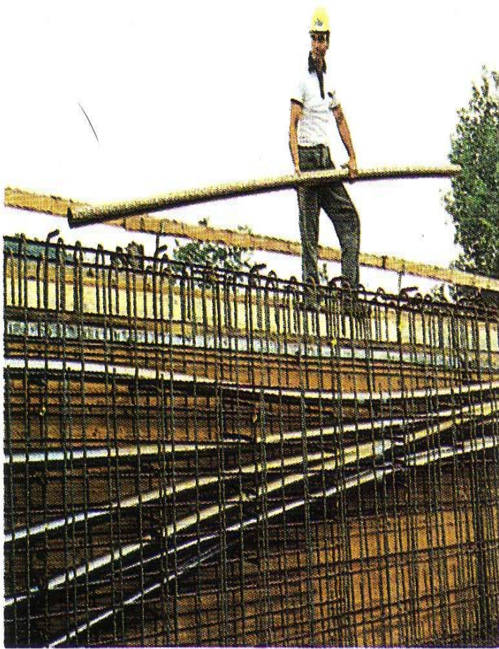
Placing of empty ducts
