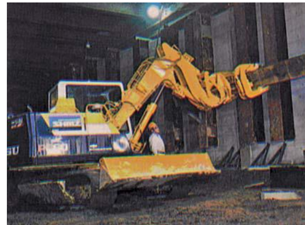
Large manipulator system (courtesy Shimizu Corp.)
