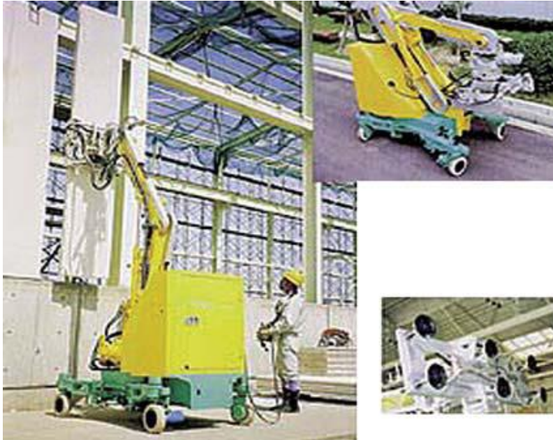
Concrete panel installation robot (courtesy Fujita Research)
