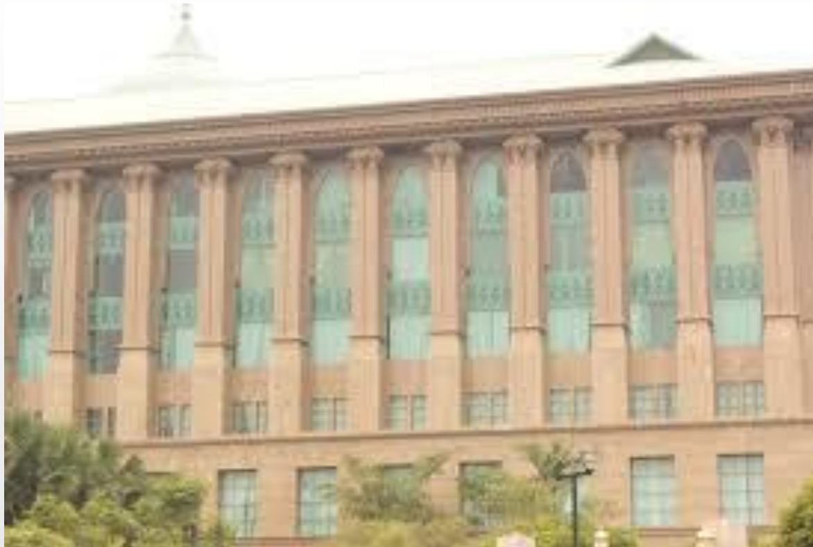
Classical columns on Malaysian Prime Minister's Office, Putrajaya
