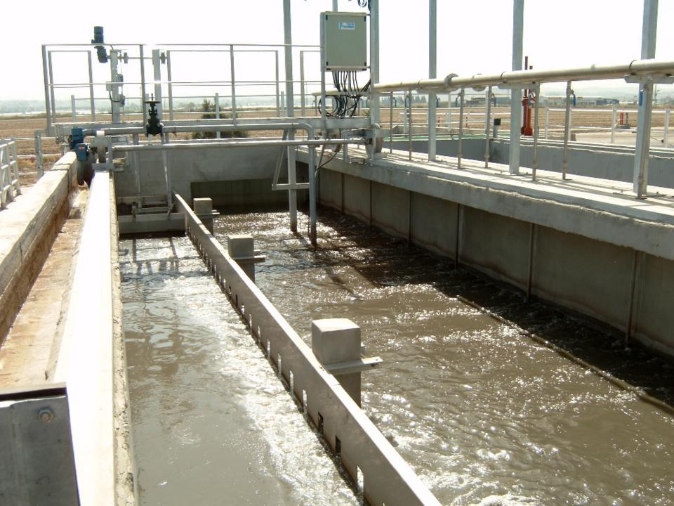
Oil and Grease Removal O & G disturb biological process Removed by floatation (skimming)
